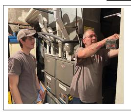
JC Heating, Cooling, and Plumbing from Gibson City installed the new dehumidifier onto the furnace on Wednesday, May 7<sup>th</sup>. It is mounted on the wall of the furnace room. The dehumidifier will reduce the percentage of humidity in the church to decrease the growth of mold especially in the rafters of the church. The dehumidifier was approved at a special congregational meeting in March and this bid was chosen by the council from the bids that were researched.
